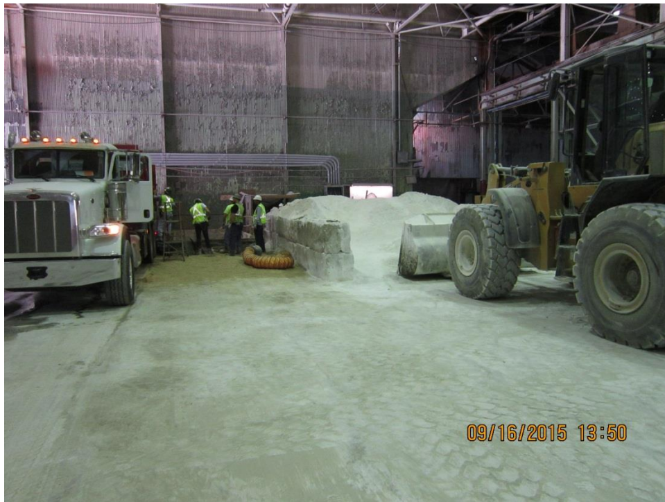
Solidification area for mixing solids with lime
