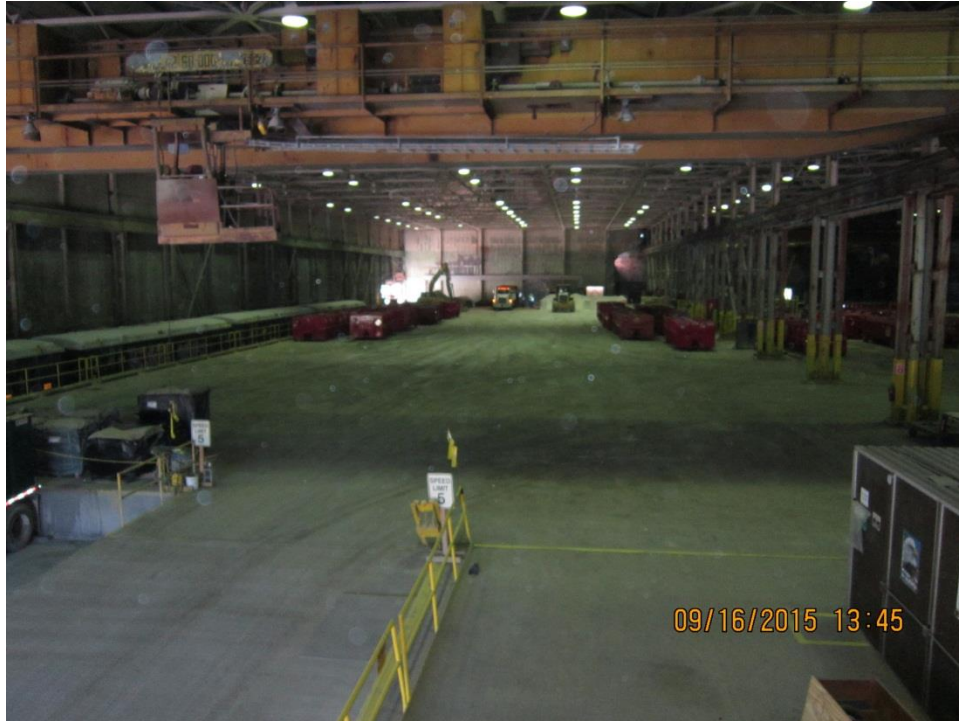
Inside of facility from office above truck entrance.
