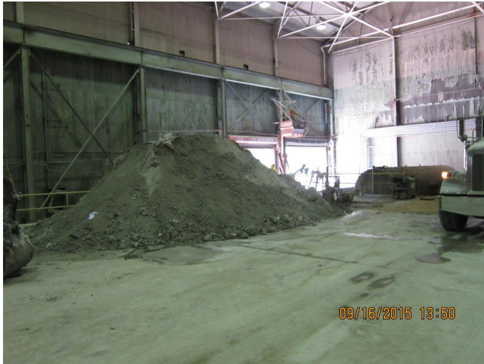
Down blended clean material ready to be shipped to West Virginia landfill.
