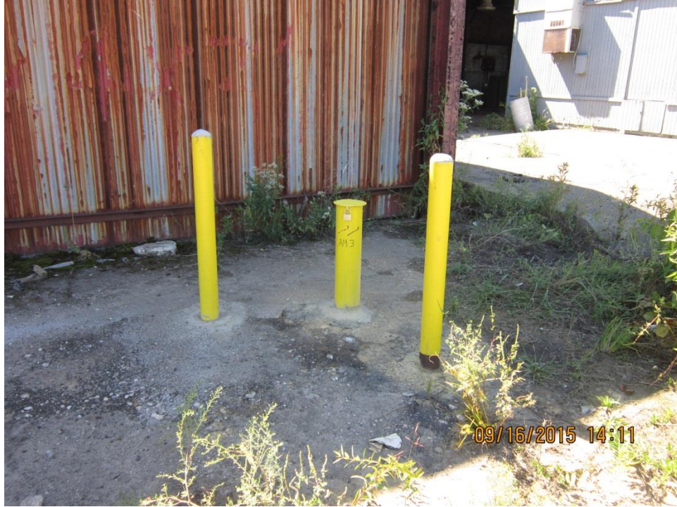
One of several monitoring wells located outside and around the facility.
