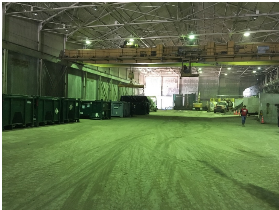
New steel boxes for disposing waste. Note that waste is not on the floor.
