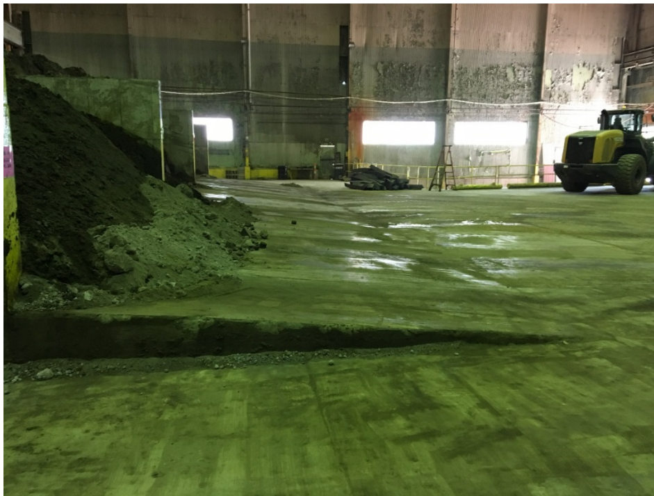
Excess waste not within containment.
